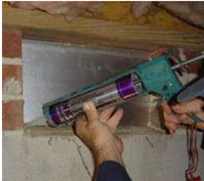
Seal holes leading to the outside in foundation walls
